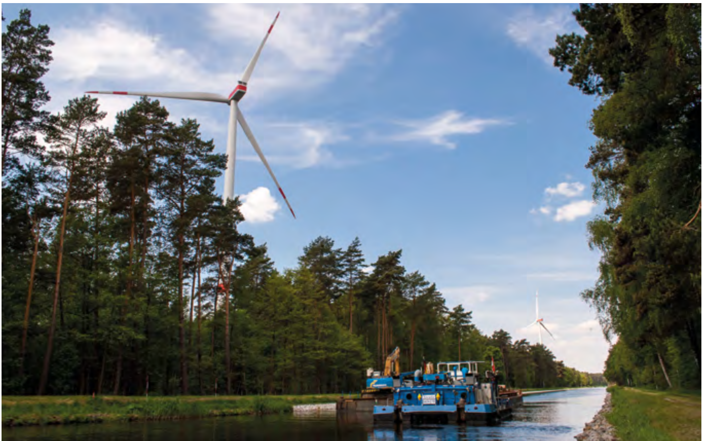
Uckley Wind Farm, Germany
