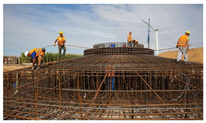
Construction of the foundation for the Wennerstorf wind farm in Germany: In this repowering project, four older turbines were replaced by two modern ones. With the two 4.5 megawatt Nordex N149 generators, the new wind farm produces three times as much electricity as its predecessor.
