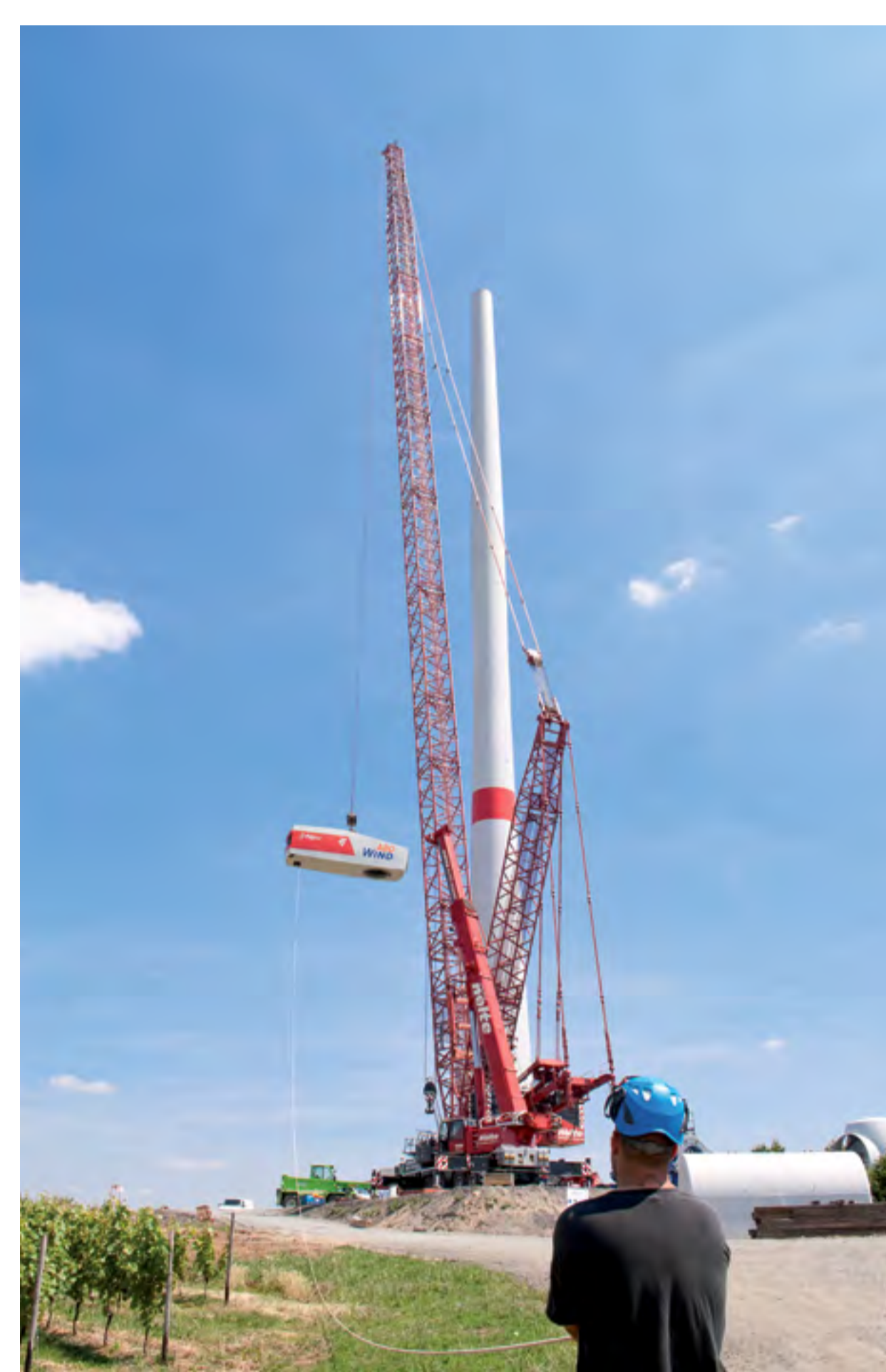
Mounting of the nacelle
