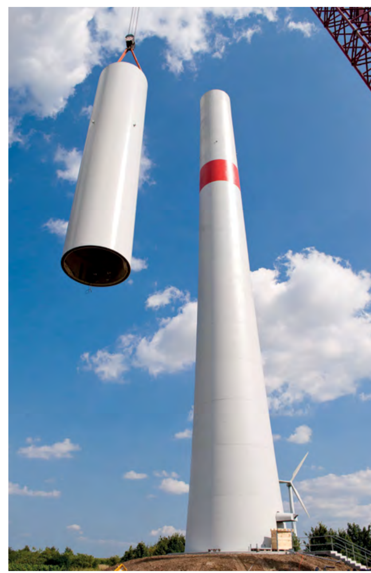
Steel or hybrid tower (bottom: concrete, top: steel)
