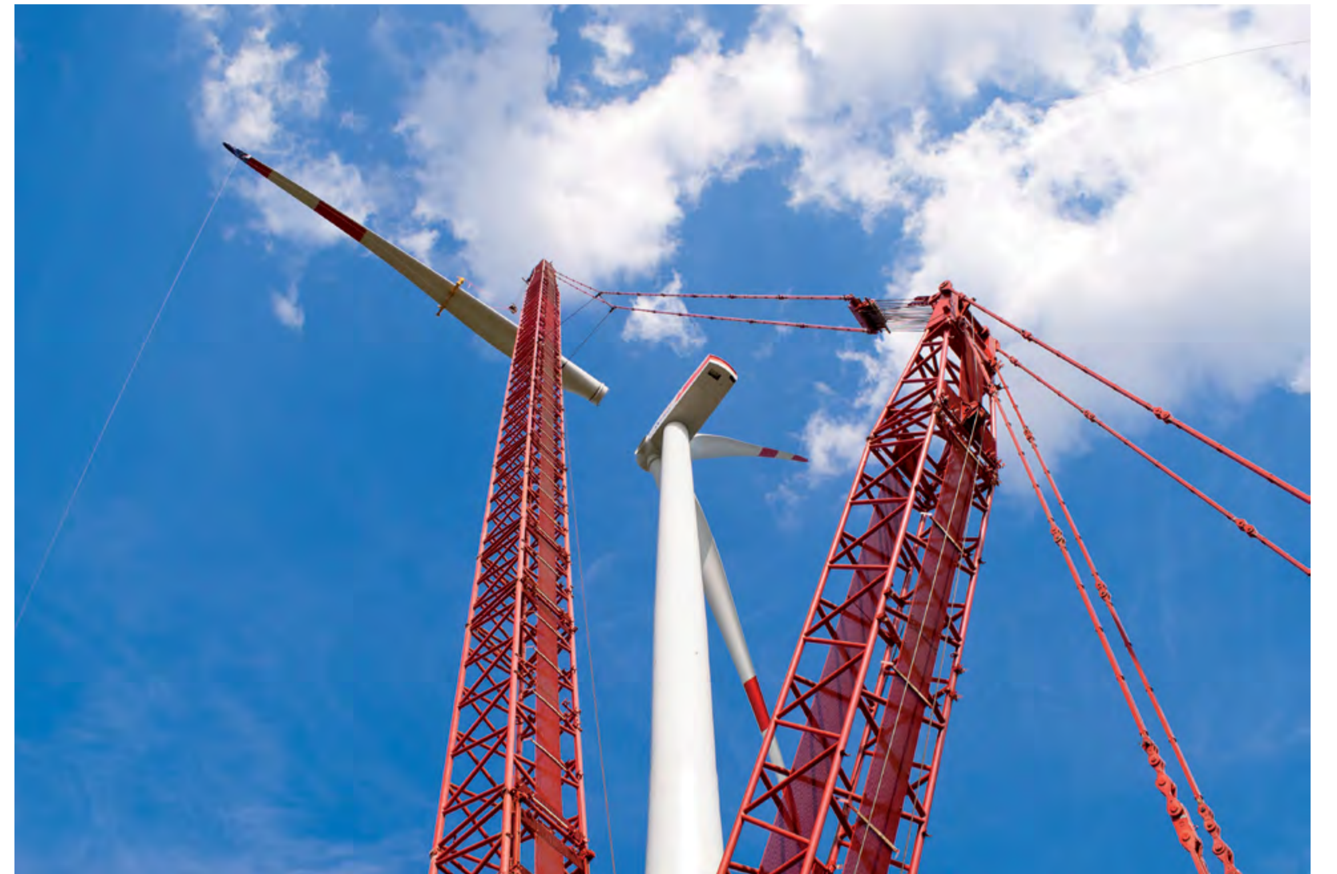
Installation of rotor blades (individually or after assembly on ground)
