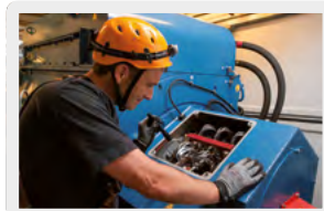
Here the technician checks the slip ring transmission on the generator.
