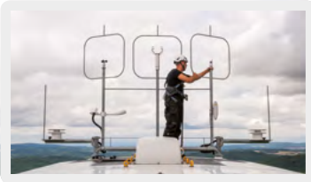
Technicians regularly inspect the anemometer, wind vane and obstruction lights on top of the nacelle.
