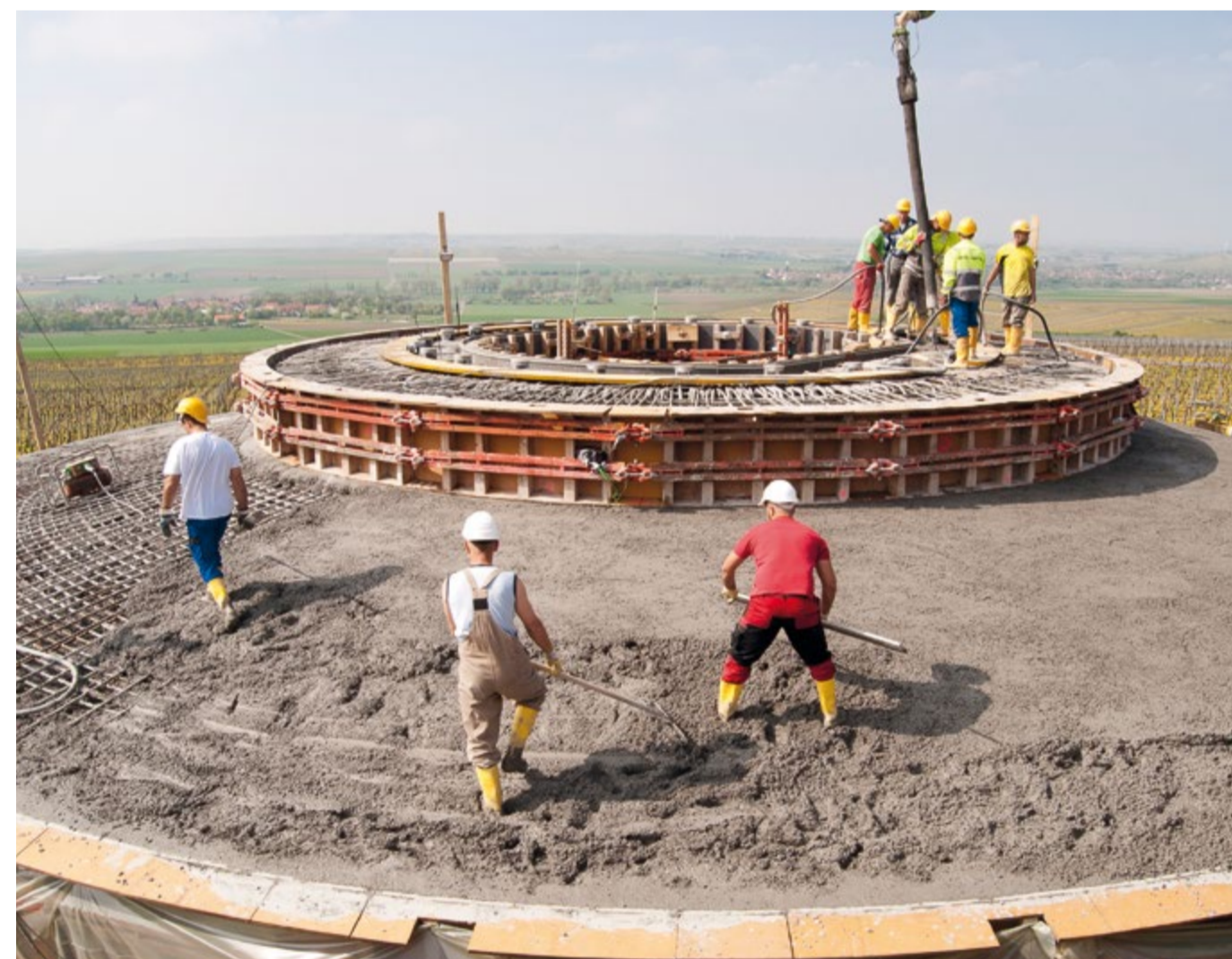
Before the turbine can be erected, a foundation is built
