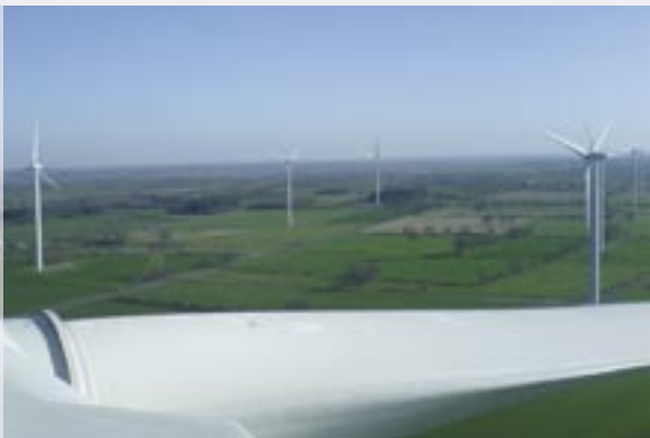
Windpark Lusanger / Lusanger wind farm
