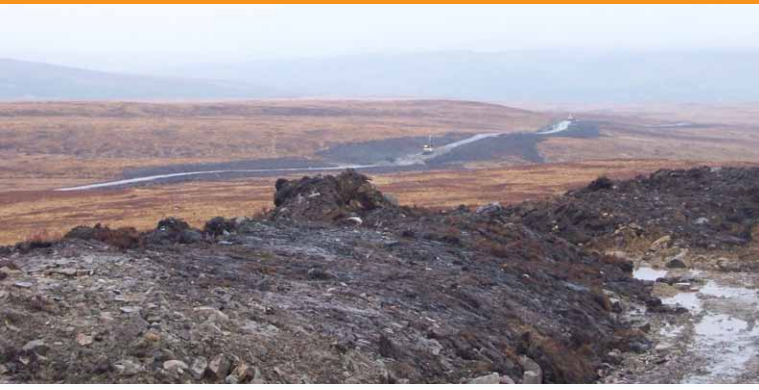
Access route under construction
