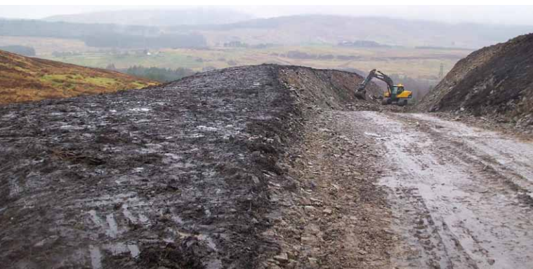
Top cut with peat reinstatement
