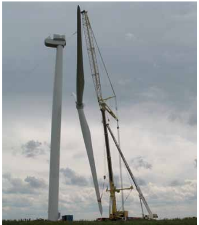
Erection of a Nordex N-80 turbine
